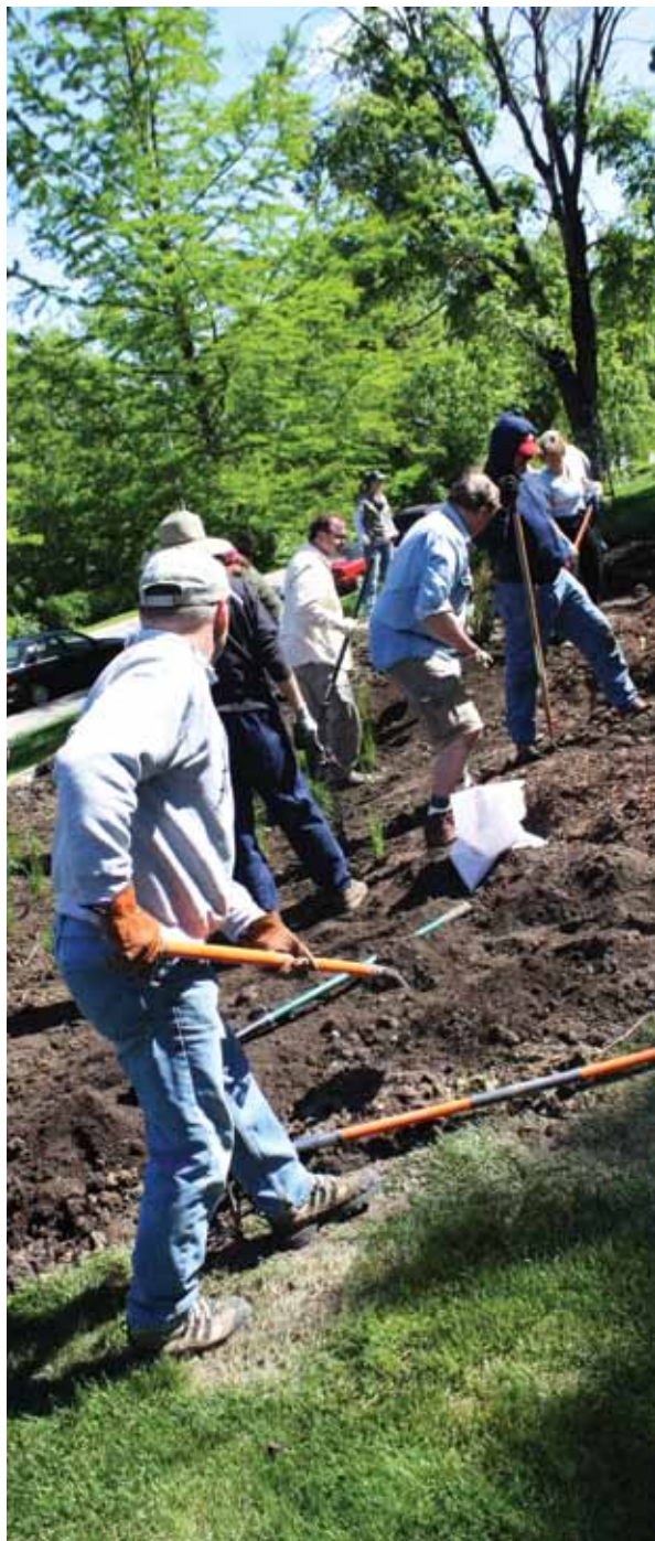
Volunteers with Sowers of Sustainability have installed several rain gardens in the zone. Rain gardens not only beautify neighborhoods but also help manage stormwater runoff.
